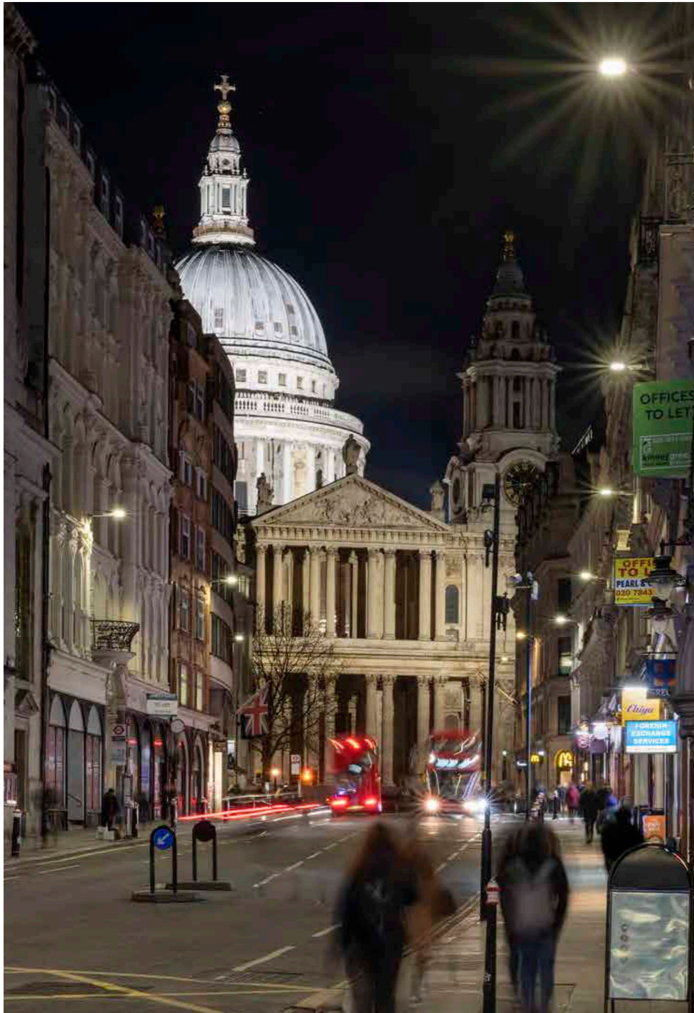
Existing lighting of St Paul's Cathedral viewed from Ludgate Hill.
